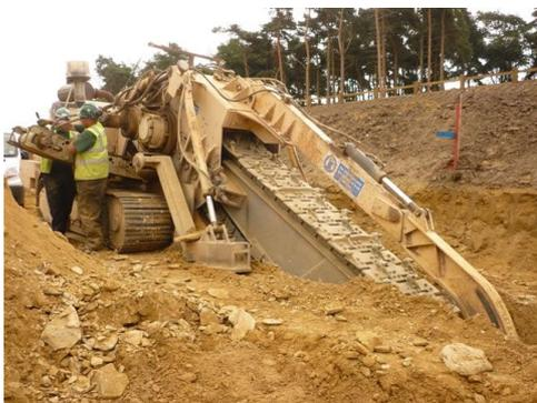
The excess excavated material from SLIN is suitable for recycling and is being taken to the quarry. The rest of the material has been used to re-contour the site and banks.
