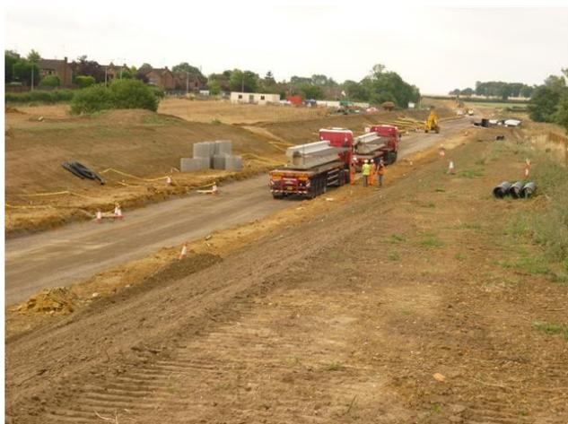
Storm water drains, or batter drains, will take water from grass slopes of the cuts of the road allowing the rain water to flow into the filter drain in the carriageway verge. These are now complete and we are just finishing off work on the filter and carrier drains throughout the site.
