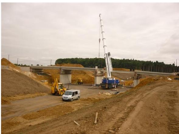
The cutting of the new road has now been completed and the next stage has started. A fantastic piece of machinery is cutting precisely the width and depth we need and as this progresses we start filling with stone. This material is a blend of 50% granite and 50% recycled tarmac planings, which are brought in daily. To date we have laid approximately 6000 tonnes of this material.
